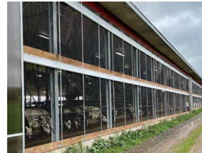
Roll up Curtain Ventilation
