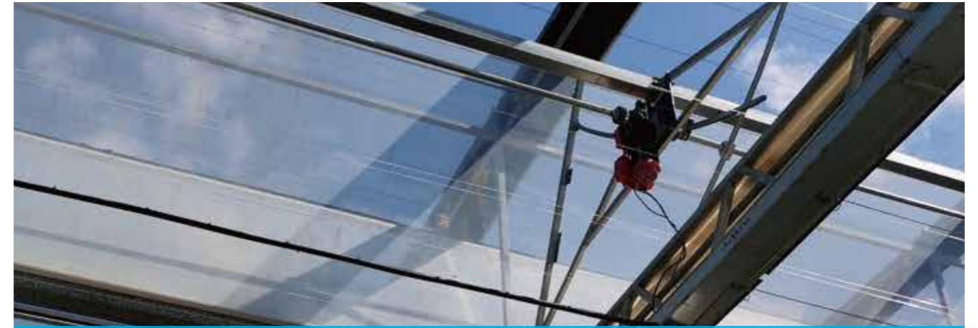
Rack and Pinion Roof Vent system
