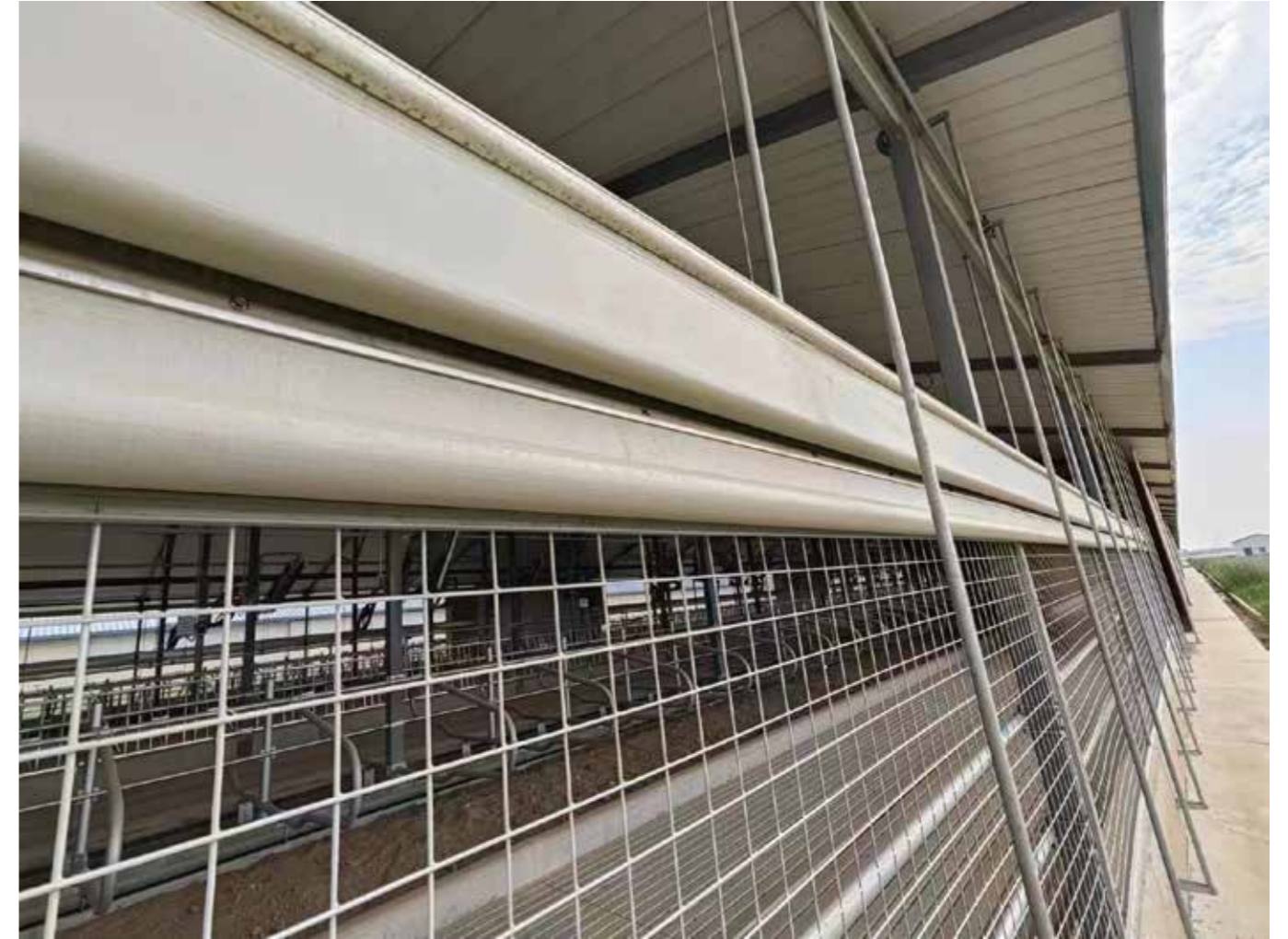
Roll over Curtain Ventilation
